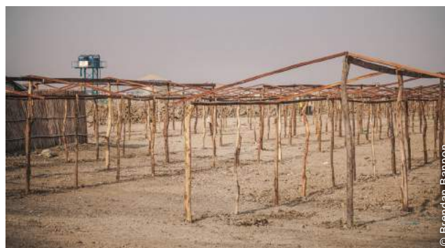
Shelter frames were built by contractors.
